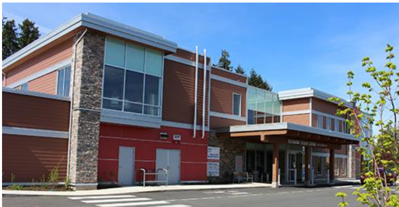
Figure 6: Oceanside Health Centre
