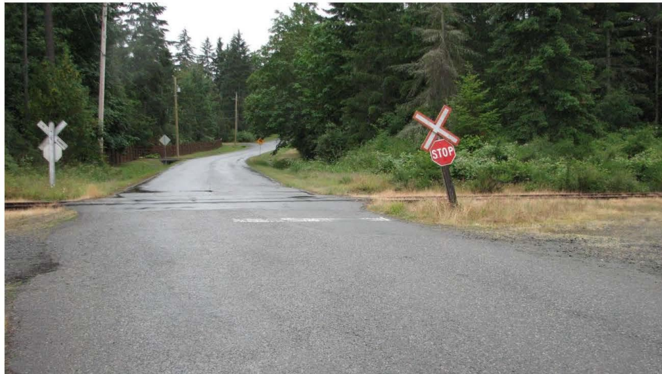
Railway crossing on Sanders Drive – Property is located to left down the tracks.
