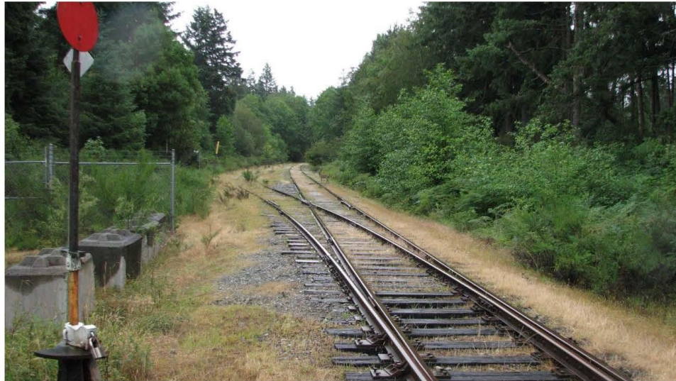
Looking down railway tracks towards subject property – a 5-7 minute walk from this point.
