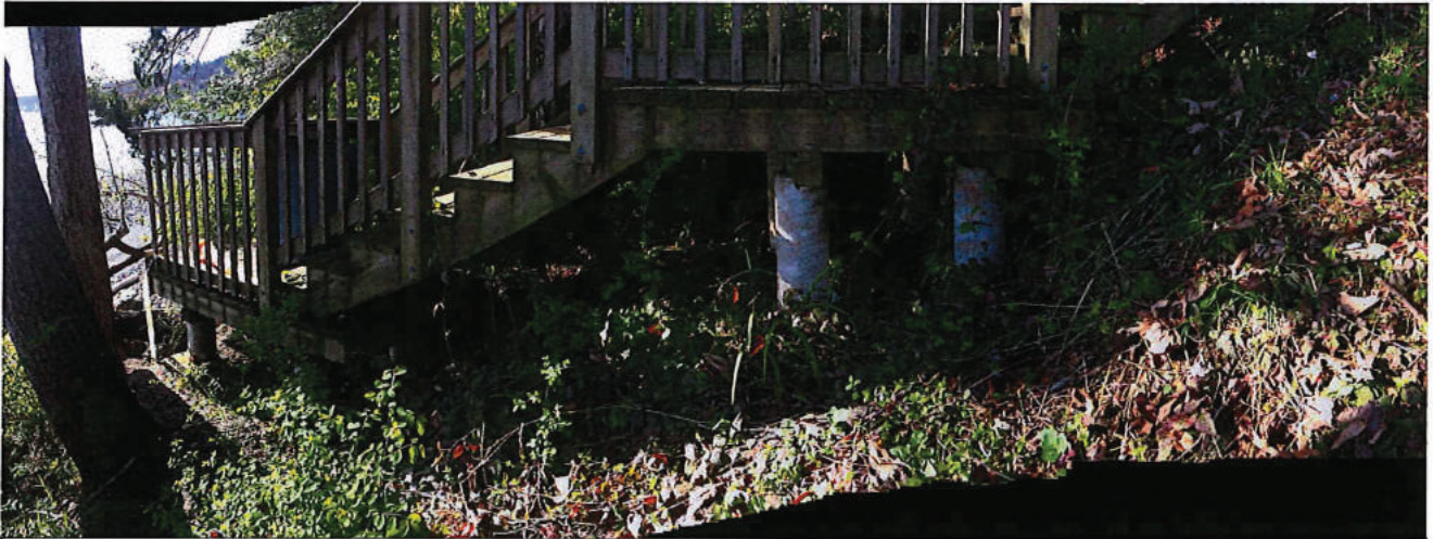
Photo 1 – Looking southeastward at beach access stairs
