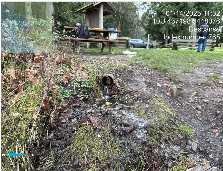
Photo 2: A drainage pipe has been installed below the parking area that conveys water from upstream drainage to the foreshore area. January 2025.
