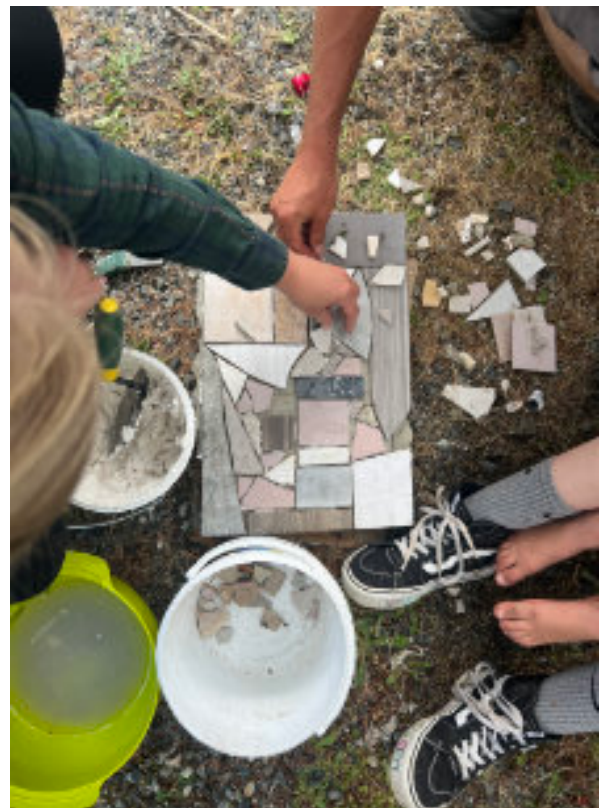
Garden paving slabs from broken tile
