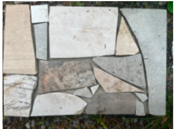
Garden paving slabs from broken tile
