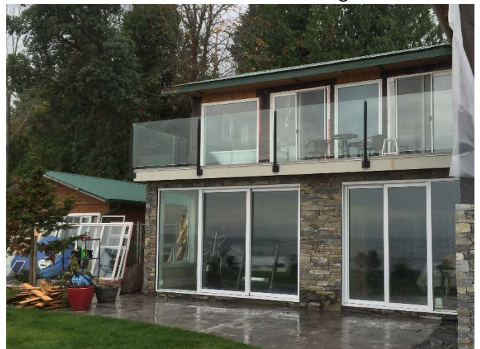
Deck Addition on October 21, 2015
