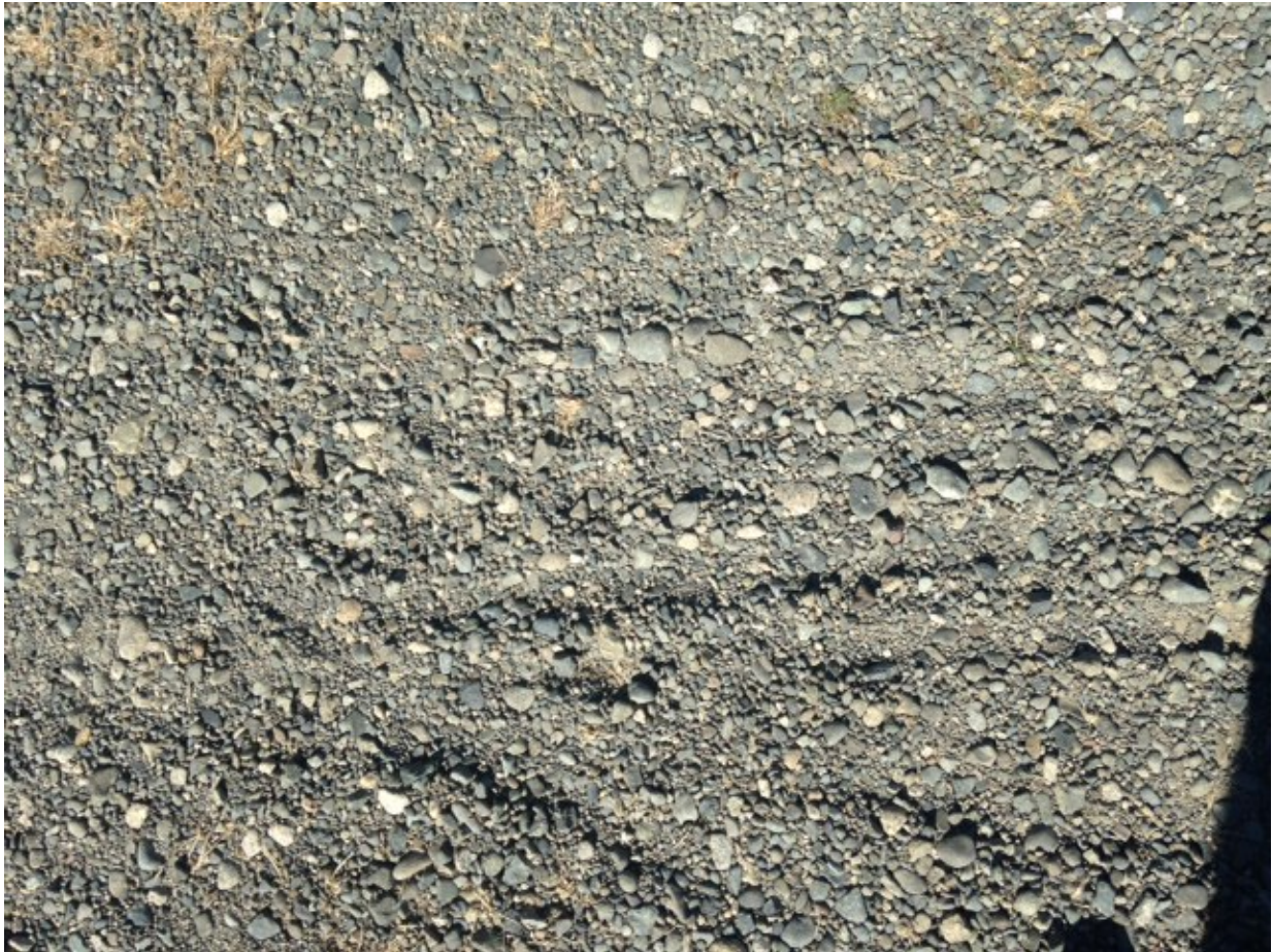
Close up of the existing surface material - rounded stone simply don not compact and are a hazard to any standard bike tire size.
