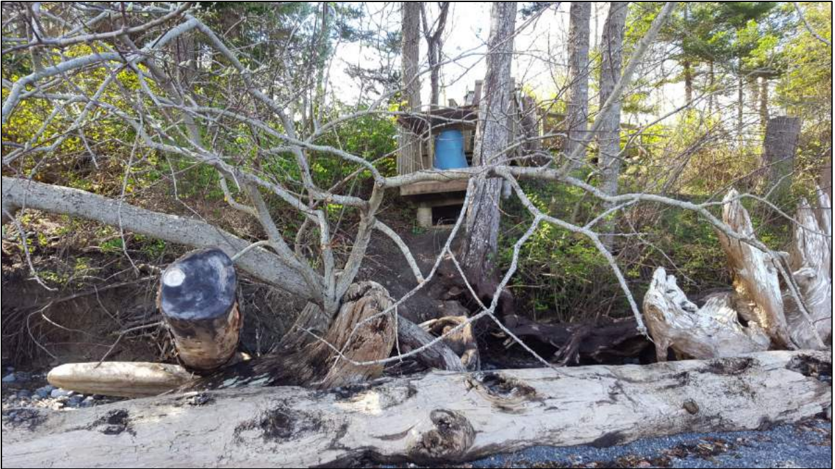
Photo 1. Looking directly at the stairs.
