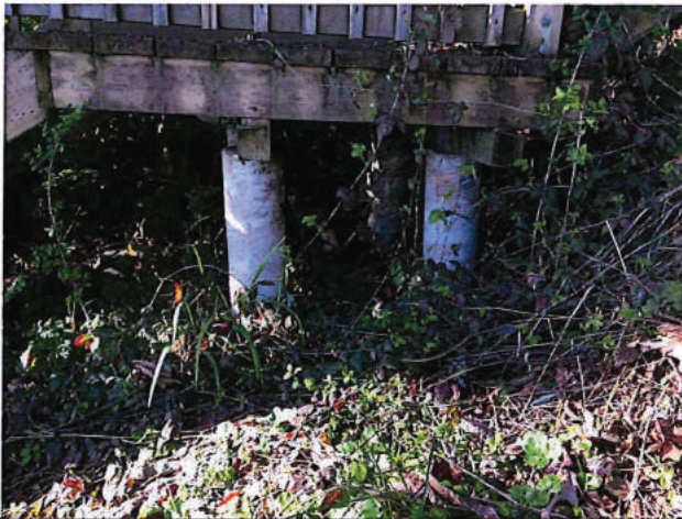
Photo 2 – Concrete pier foundation on upper slope
