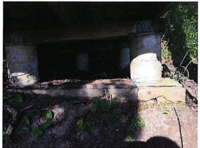
Photo 4 – concrete pier foundation on lower slope
