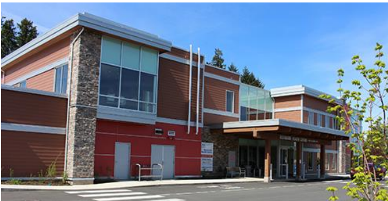
Figure 6: Oceanside Health Centre
