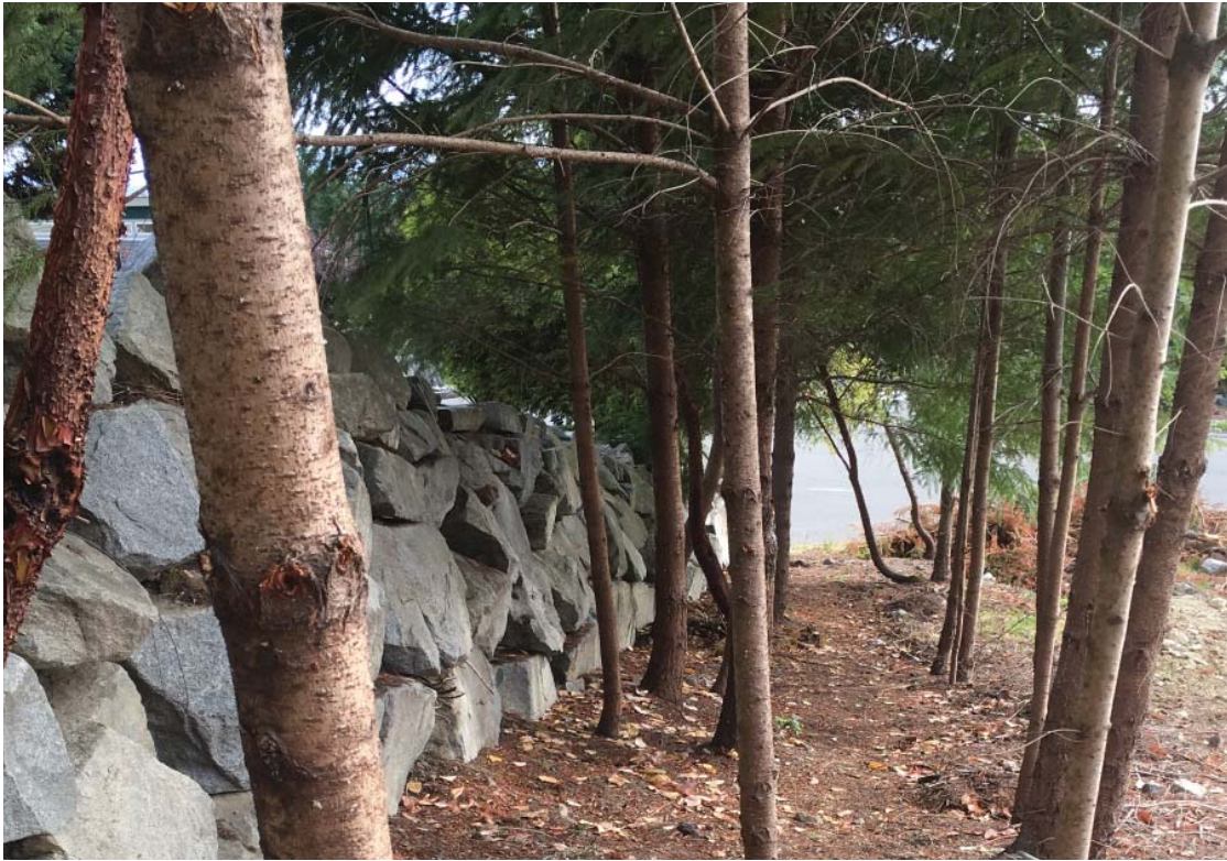
Image 5 (above): Small group of regenerating evergreen trees. One or two small diameter trees would require removal to open up walkway. Compatibility with underground infrastructure to be confirmed.
