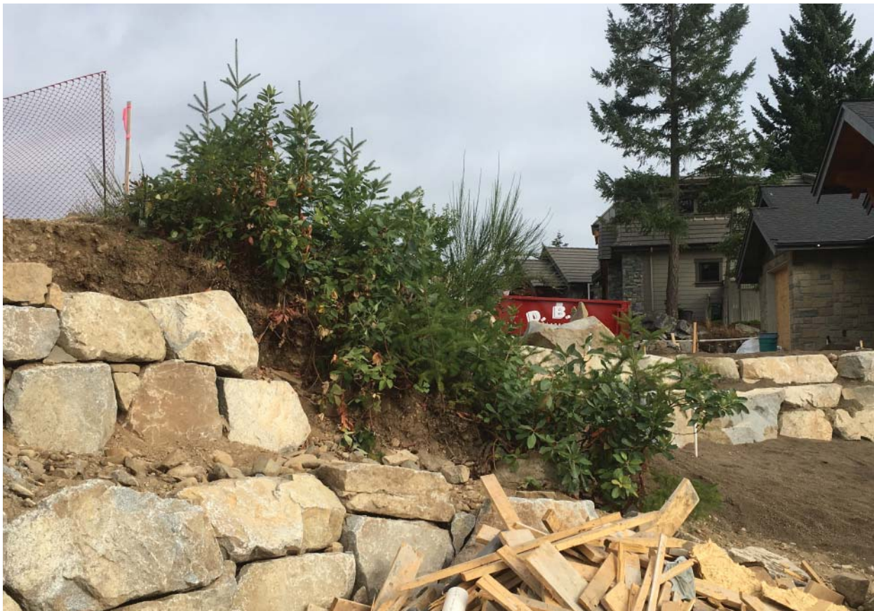
Image 2 (below): Approximate 2m grade change (existing vegetation) that would require bank retention and stairs. Adjacent bank retention by neighbours visible.
