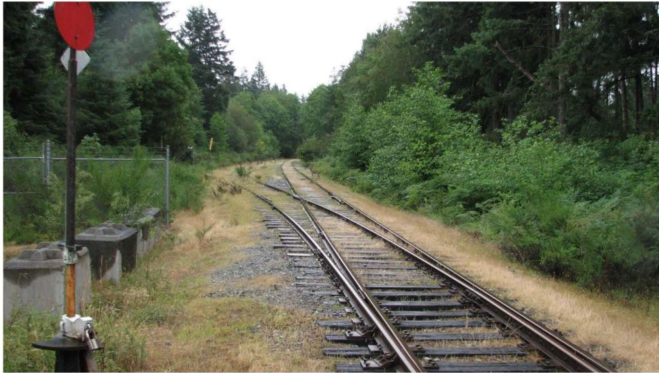
Looking down railway tracks towards subject property – a 5-7 minute walk from this point.
