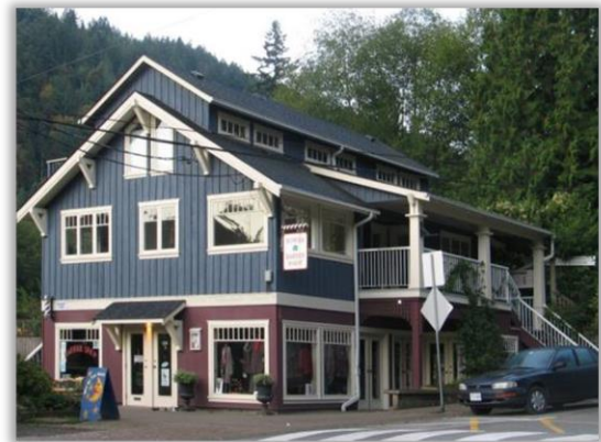
Example of mixed-use building with third floor roofscape.
