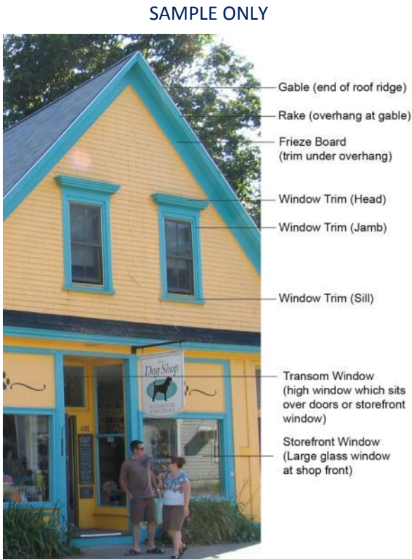
Illustration showing the use of frieze boards and other trim
