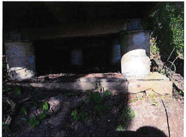
Photo 4 – concrete pier foundation on lower slope
