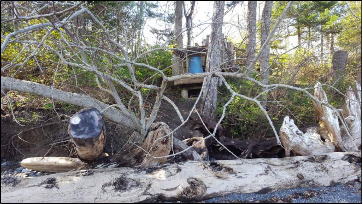
Photo 1. Looking directly at the stairs.
