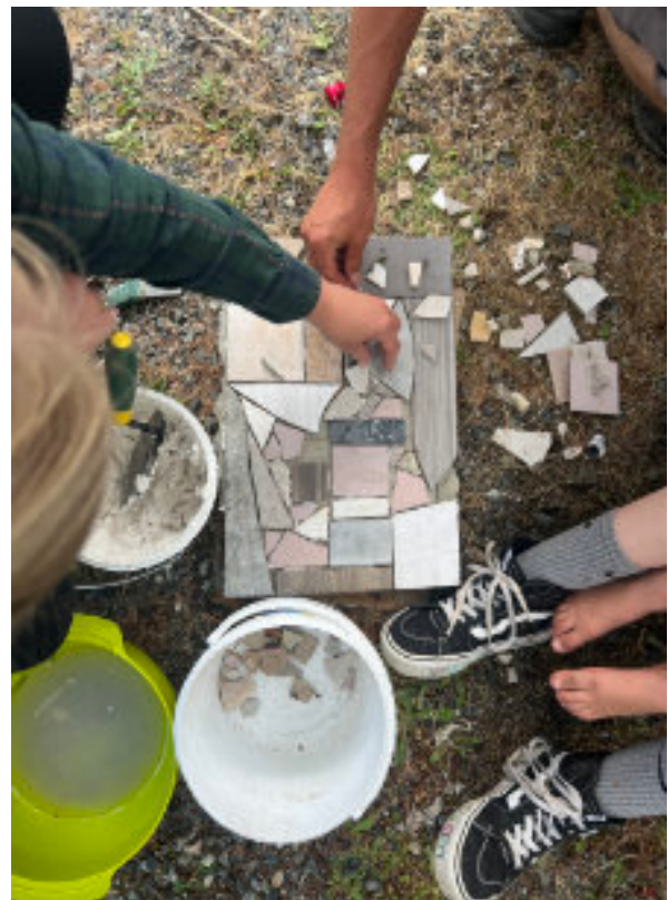
Garden paving slabs from broken tile
