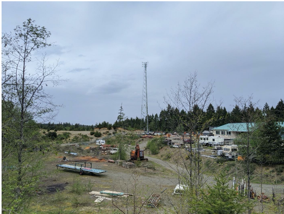
2 - Northeast Elevation - View Looking North from Subject Property (for discussion purposes only)
